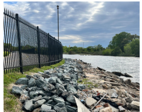
Hampton VAMC Perimeter Fence
