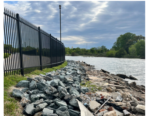
Hampton VAMC Perimeter Fence
